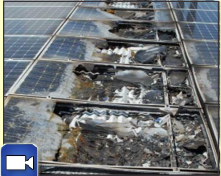
AFCI listed devices required by code to prevent fires
